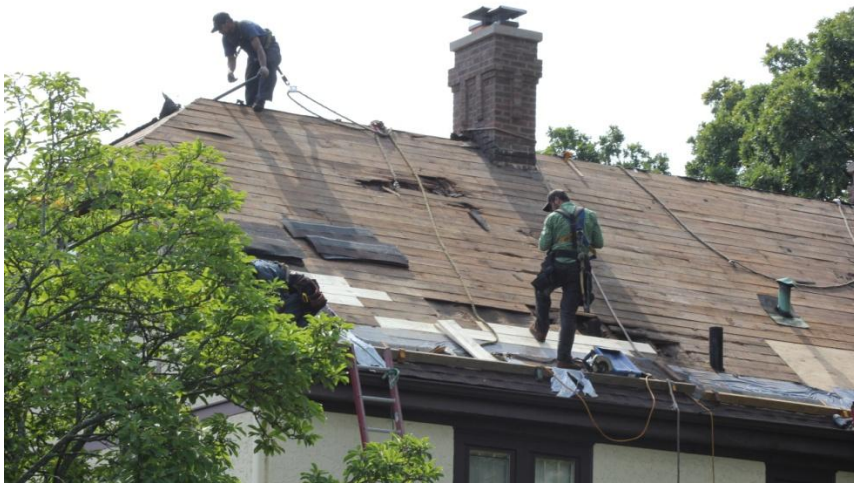
Figure 5. Workers in PFAs on a 10:12 pitched roof.
