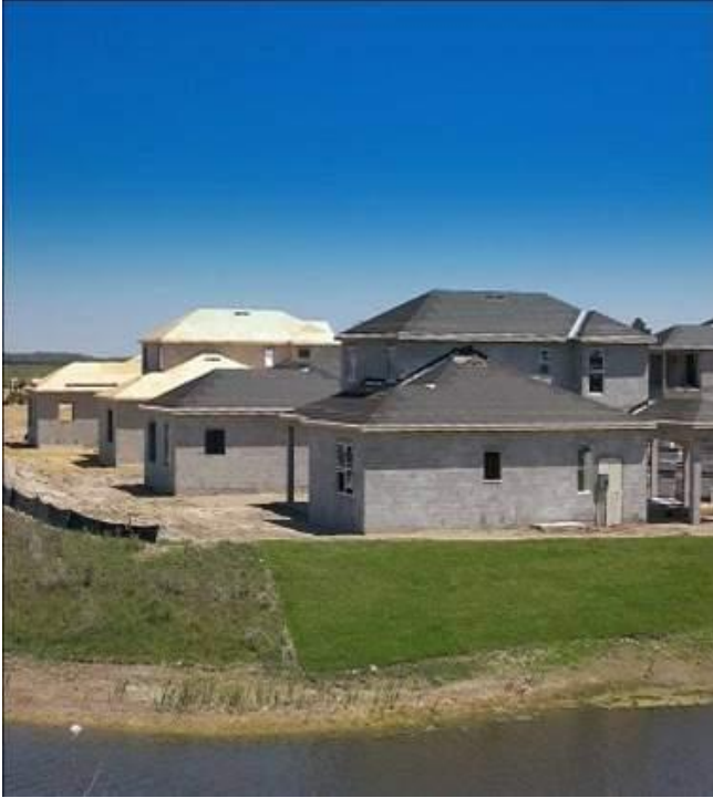
Figure 6. A typical new, residential construction work site.
